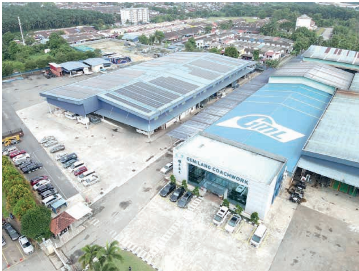
Photo of the Photovoltaic System in the Manufacturing Plant
